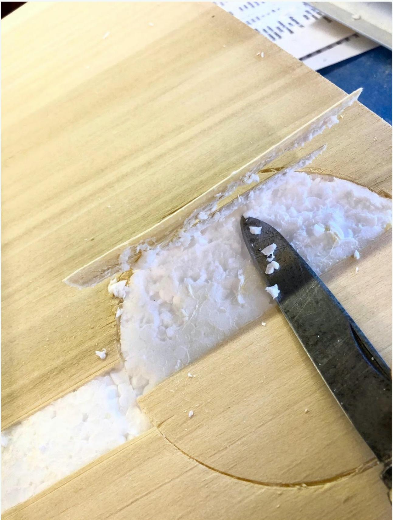
and used the soldering iron to remove the foam.
