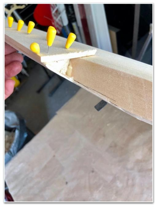
Pictures are worth a thousand words and I think this one shows what I mean. I was then able to form a better profile and then was in a position to glass the wing join using epoxy resin. The next shots show how the balsa 'filler' pieces have been sanded back to give me a more pronounced forward taper.
