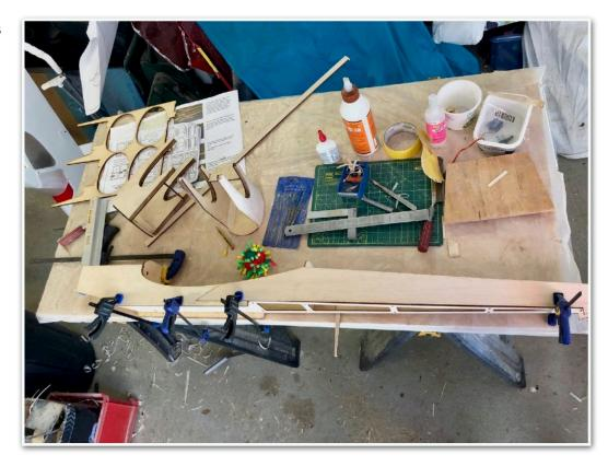
Tail pulled in, clamped and pinned.
