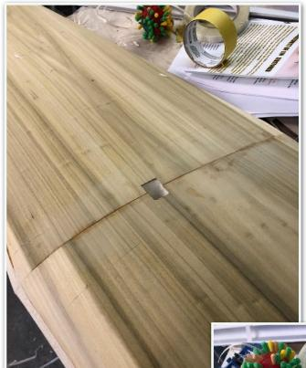
And then the joint was reinforced with glass cloth and epoxy resin.
